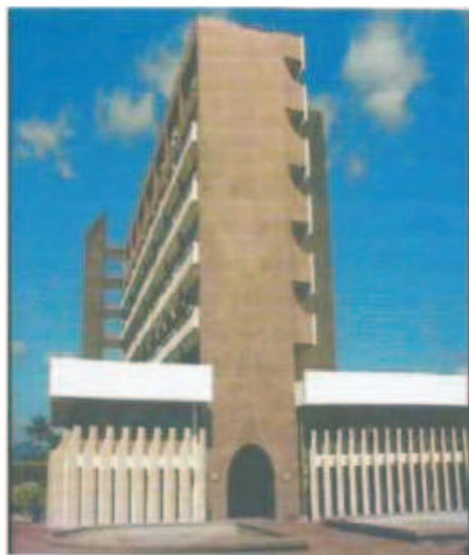
Approach Elevation of the OAU Senate Building. Source: Author's Field Survey, 2017
