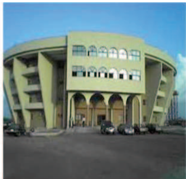
Approach view of LAUTECH Senate Building Source: Author's Field Survey, 2017
