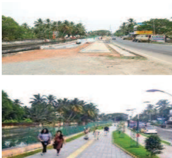
Figure 1: The Streetscape Project During Construction And After
