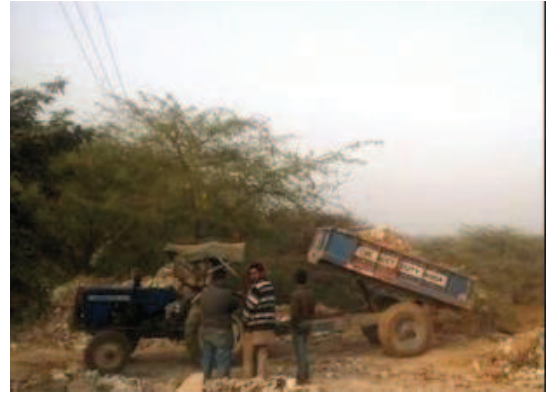
[Actual site photographs taken by the authors]
